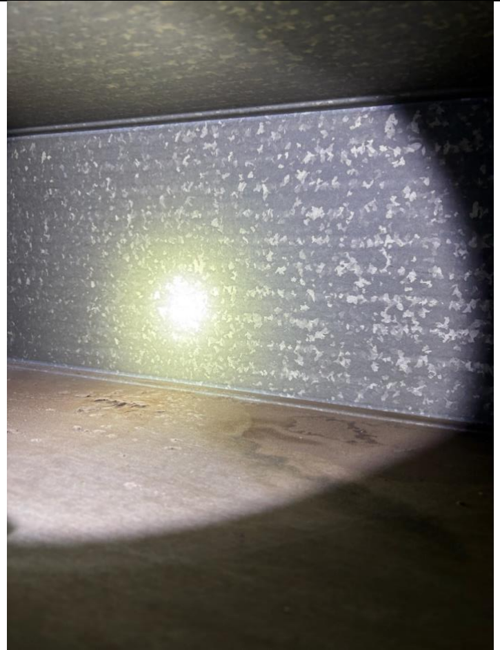
Evidence of dirt and debris on HVAC duct interior.
